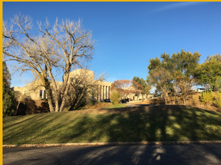
West retaining wall of south parking lot
