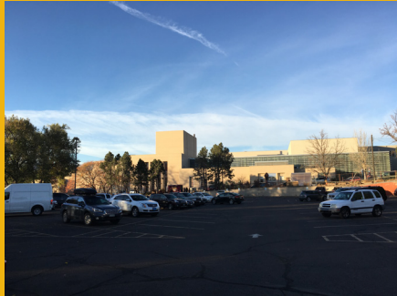
FAC facing the south parking lot
