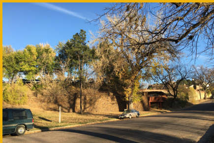
West retaining wall of south parking lot
