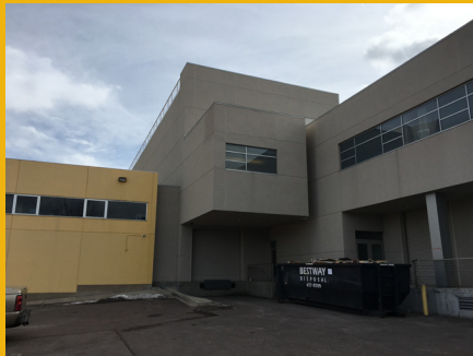
Existing FAC Loading Dock
